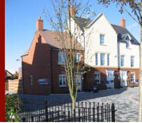
Archers Gate Housing Scheme
