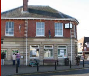
Salisbury Street/High Street Junction
